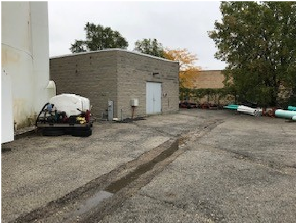
Village of Lincolnwood potable water pump station on east side of tower. Contractor to modify containment curtain to not disturb normal operations of this building.
