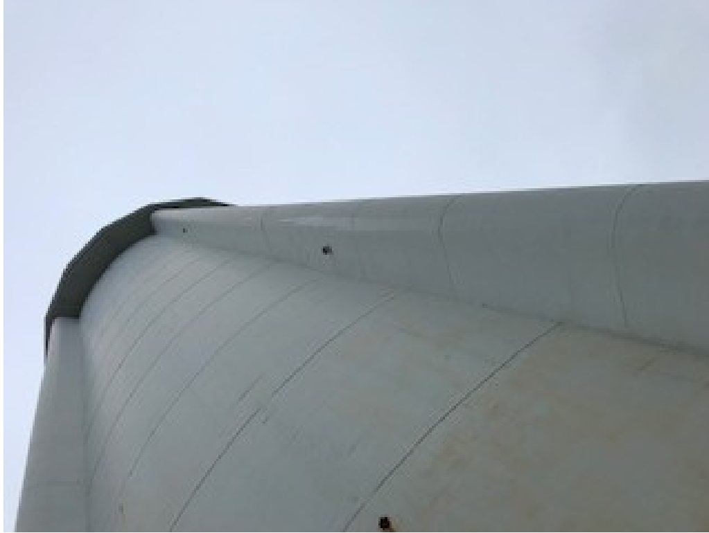
Vertical view of tank exterior.
